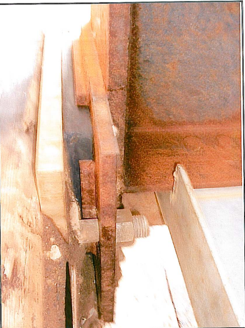
Photo 11 Anchor bolt at the south girder of the west abutment. The bolt is centered in the slotted hole.
