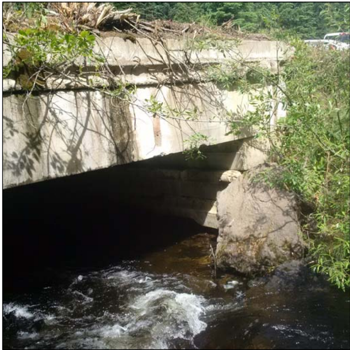
PHOTO #3 - VIEW OF STRUCTURE AND ABUTMENT
