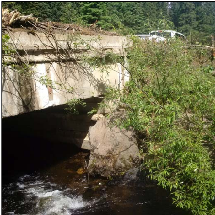
PHOTO #6 - VIEW TOWARDS UPSTREAM
