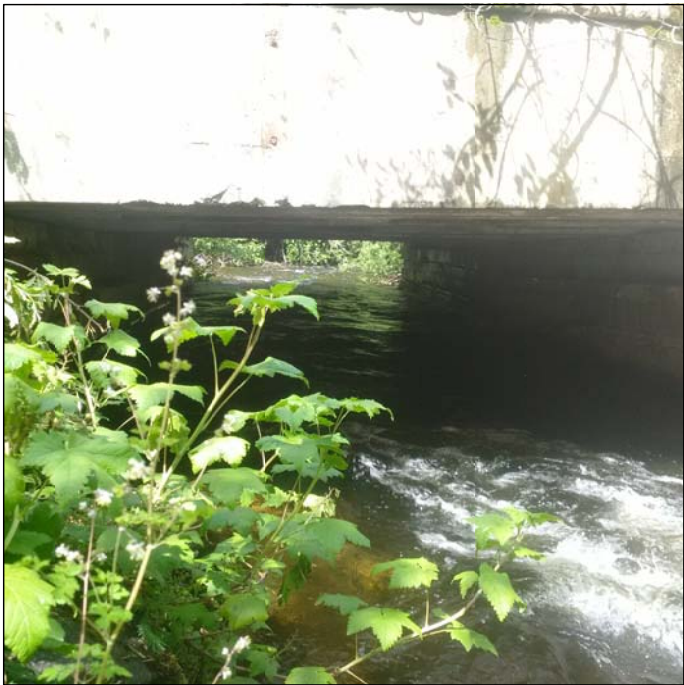
PHOTO #5 - VIEW TOWARDS DOWNSTREAM
