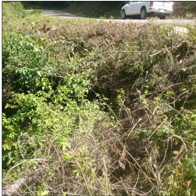
PHOTO #4 - VIEW DOWNSTREAM OF CROSSING
