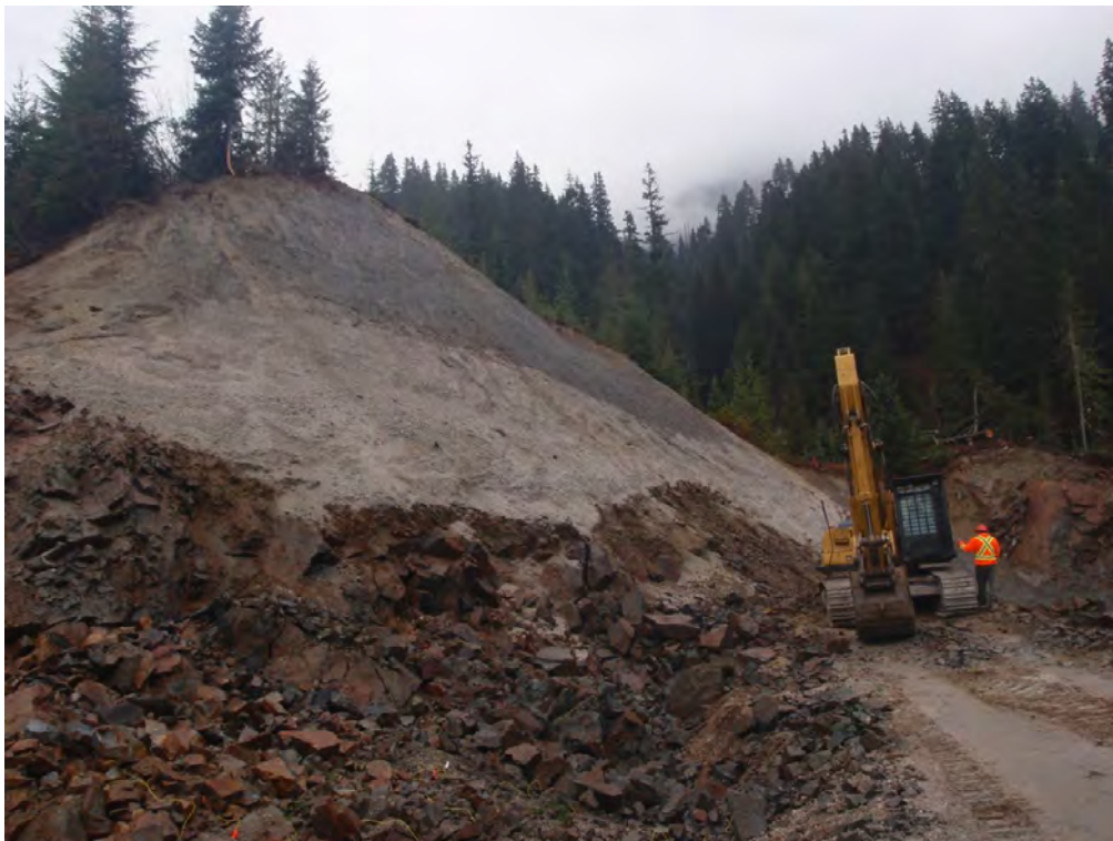
Photo 6. 35 m tall exposure of Pebble Creek Formation on the bush side abutment of the Truckwash Creek FSR bridge. Rock avalanche debris (grey) overlying tephra (white).
