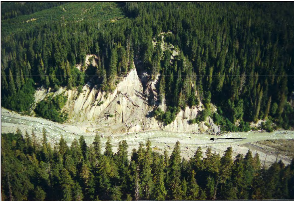
Photo 2. Bank failure in edifice collapse debris, 140 m tall and 200 m wide on the south bank of Meager Creek just upstream of Hot Springs Creek fan. Debris at the foot of slope has deflected the channel left, and sediment additions likely affect bed stability downstream.
