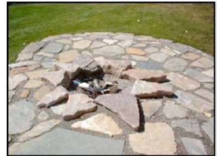
Exhibit 2.: An example of the desired type, size, texture and colour of paving stones as described by the landscape design guidelines (courtesy of Tom Barratt Ltd.)
