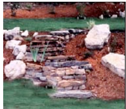
Exhibit 7.: An example of a staircase composed of assorted slate tiles (courtesy of Tom Barratt Ltd.).
