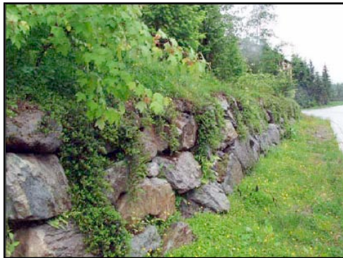
Exhibit 5.: An example of native Kinnickinnick planting on a retaining wall (courtesy of Tom Barratt Ltd.).
