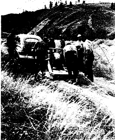
Crew laying cable as car tows cable reel up the hill.
