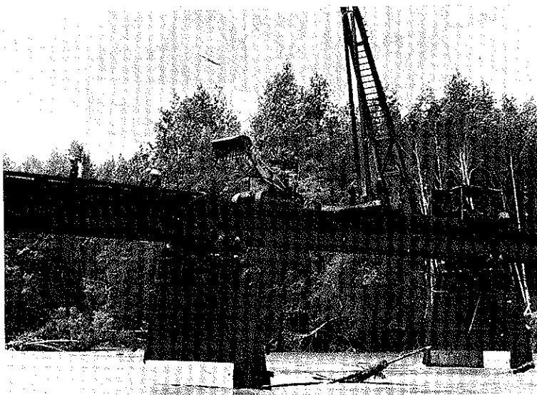
Part of the Kingcome River bridge. The pile-driver has finished its work and is being skidded by the tractor back over the bridge.
