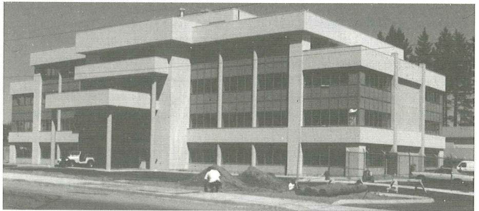
New Nanaimo headquarters for Vancouver forest region nears completion.
