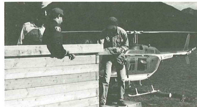
Dawson Creek forest district staff Kevin Hanna (r) , Mark Kusalik and Cliff McKay (l) work on the restoration of the Wapiti cabin.
