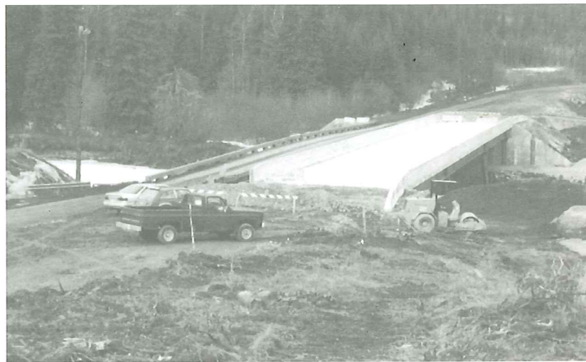
The newly completed Murray River Bridge — just over two months work for a dedicated team of Forest Service engineers and contractors.
