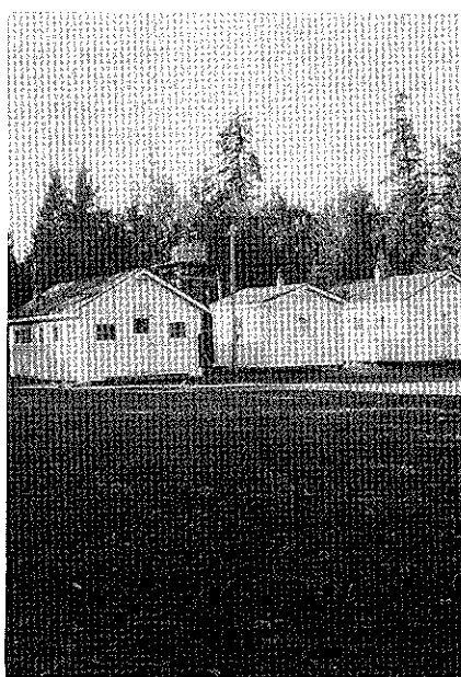
Nanaimo Suppression Camp. L. to r. Cookhouse and diningroom - Foreman's dwelling and office - Wash-house.
