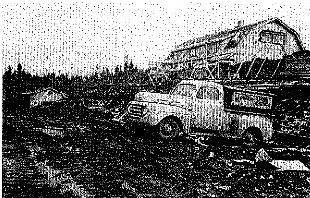
Garage, far left, and office-stores building under construction at Aleza Lake Station.
