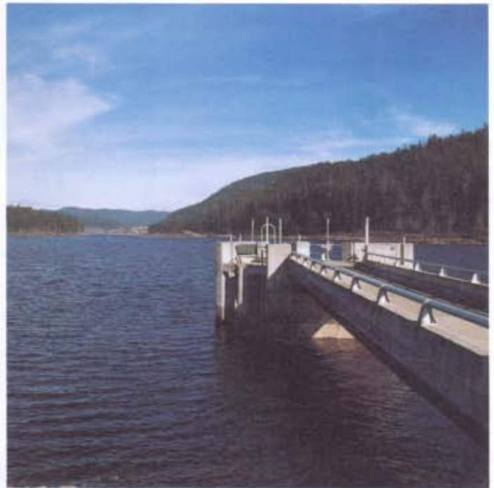
At peak periods during the summer months, Victoria water district's main intake at Sooke Lake draws out 40 million gallons of water each day to satisfy its customers.
