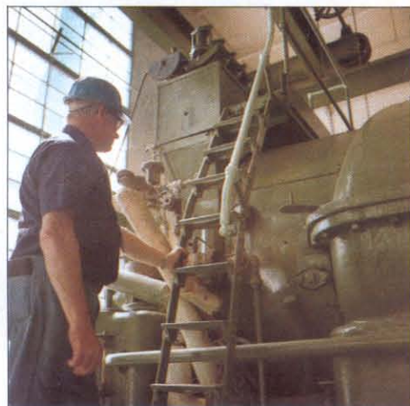
Engineer Walter Mitchell stands back from the intense heat of one of three Dutch ovens at Crown Zellerbach's Fraser Mills lumber and plywood plant. These ovens burn hog fuel and bark to generate almost all the electrical energy required by the plant.
