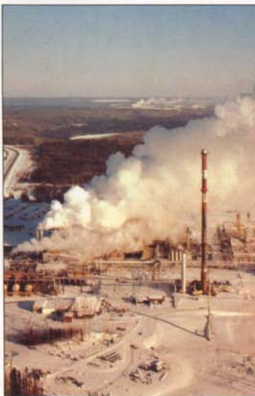
This gas plant on the outskirts of town highlights the fact that the natural gas found in the Fort Nelson area makes an important contribution to the B.C. economy. The economy of Fort Nelson itself, however, depends much more on the local forest industry, which employs eight workers for every one in the gas industry.
