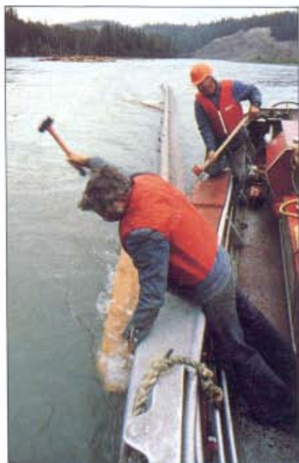
Jetboat operator Ron Wilkins (above) works on a finboom, a long, floating line of logs with one end anchored onshore. Finbooms protect sidechannels, gravel bars and river banks from the full force of the logs as they head downriver. The Quesnel is a salmon river, and there is a bare three-week interval between outward and inward salmon migrations in which to get the logs moved. That three-week period is established by the federal department of Fisheries and Oceans. Critics of the log drive claim it has damaged fish habitat and lowered fish population levels in the river.
