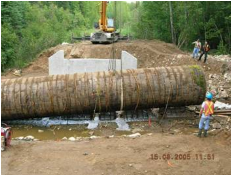
Our first attempt to lift the culvert in one piece. It was too heavy, but our hopes were definitely raised with how solid it appeared. We really believed it was going to happen at this point.
