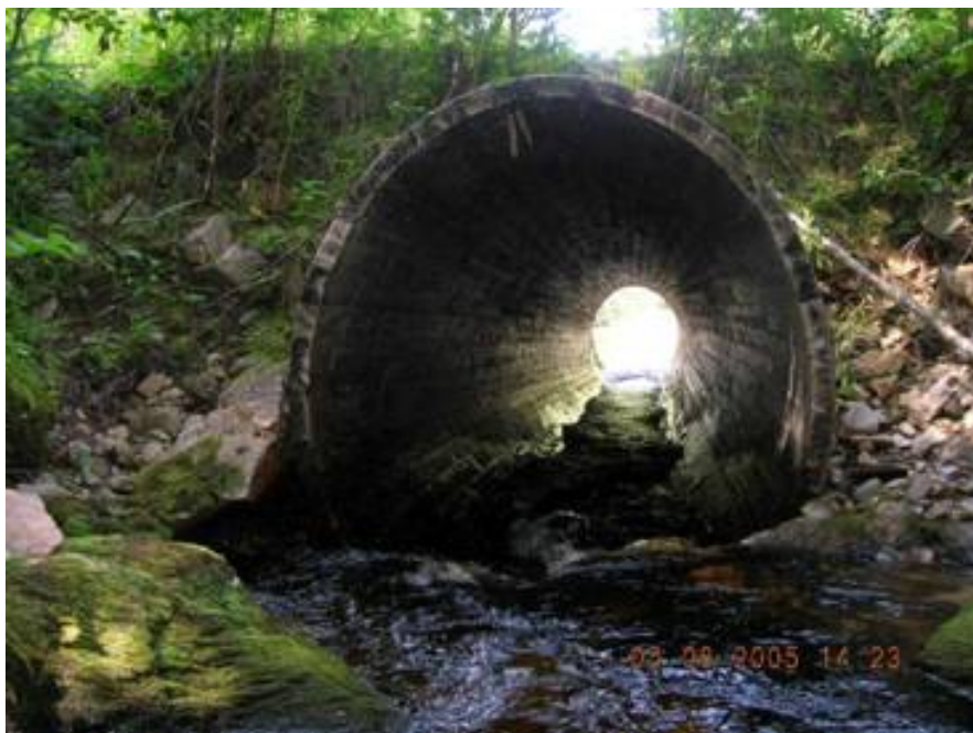
The inlet of the culvert about a week before we started the construction.
