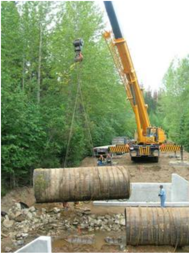
The first 6-meter section successfully lifted to the awaiting lowbed for its trip north.
