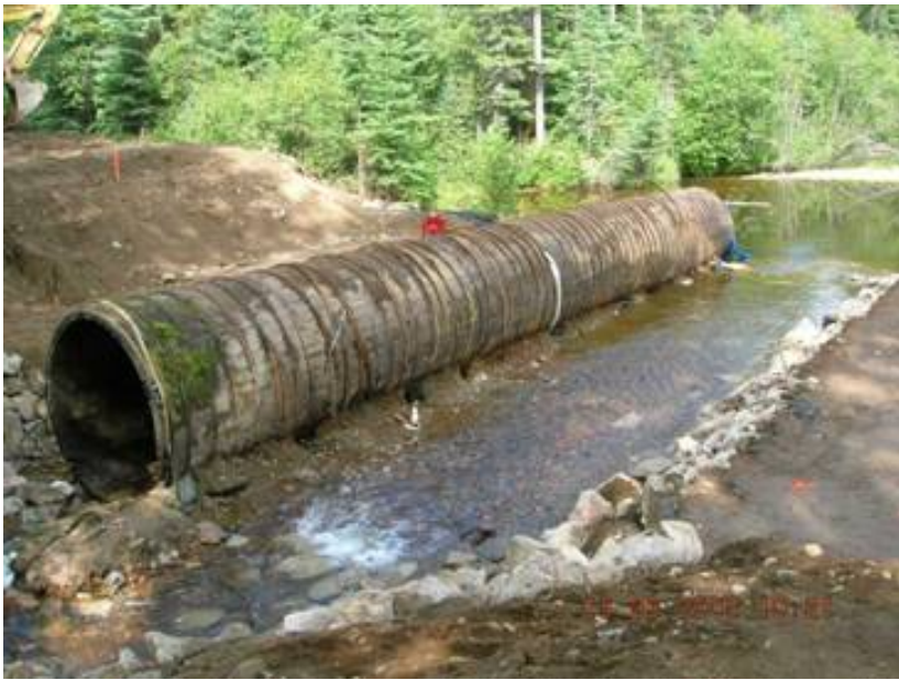
The entire culvert with the original banding in place.
