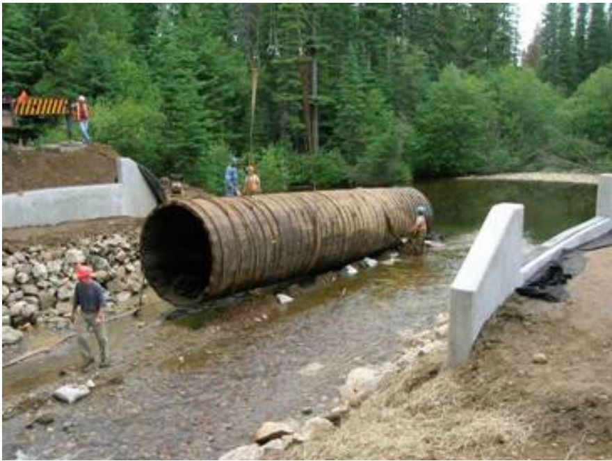
The second 12-meter piece being successfully lifted from between the abutments for the new bridge.
