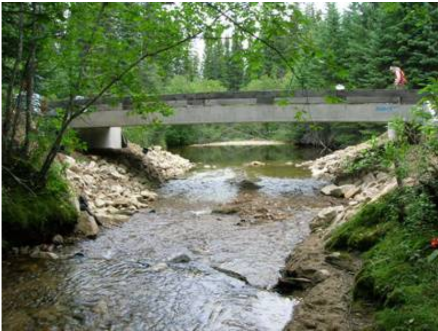
The new concrete slab girder bridge that was installed on the site.
