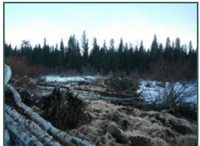
Figure 2. Aspen barriers were placed along and perpendicular to the stream to create cells.
