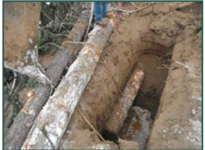
Figure 4. Anchoring conifers into the streambank.
