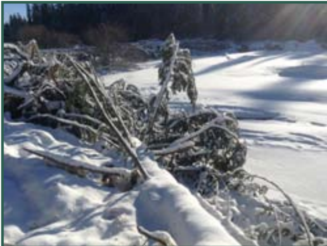
Figure 5. Conifers anchored into the streambank.
