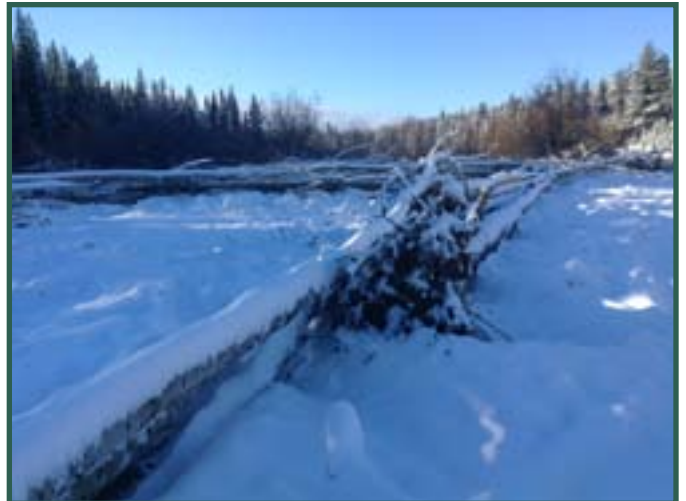
Figure 6. Aspen tree barriers protecting the streambank.
