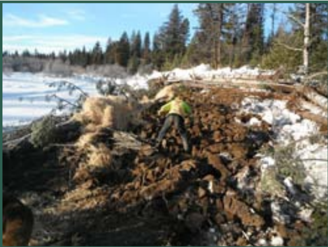
Figure 3. A Baker Creek Enhancement Society worker inserting willow whips in loosed soil next to stream.
