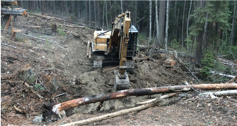
Excavator ensuring that natural drainage patterns are maintained post-wildfire. Canim Lake Wildfire (Cariboo Fire Centre)
