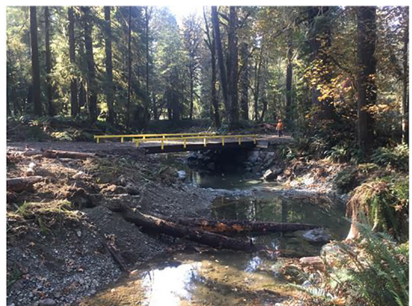
Bridge installations complete.
