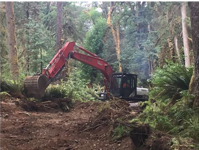
August 2020 – Channel excavation begins
