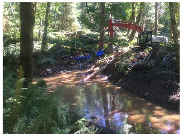
Channel and bank grooming; placement of original revegetation
