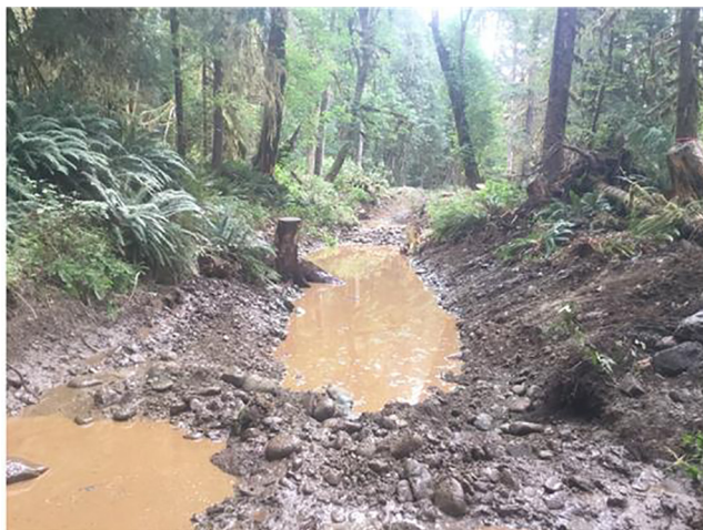
Channels brought to required elevations.
