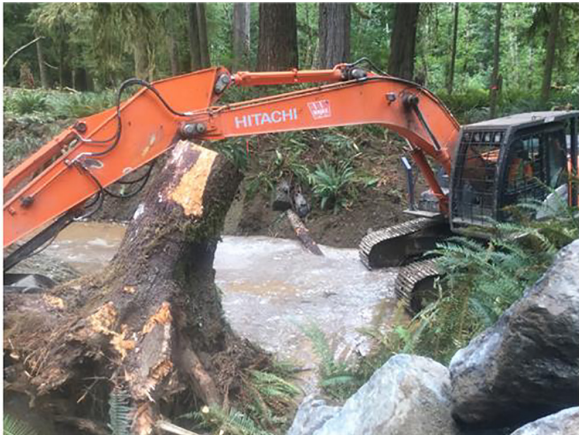
Channels complexed with the addition of woody debris and boulders.
