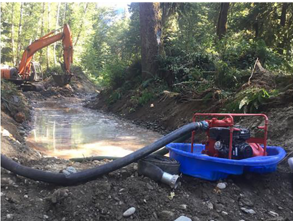
Typical sediment control measures used for the project.
