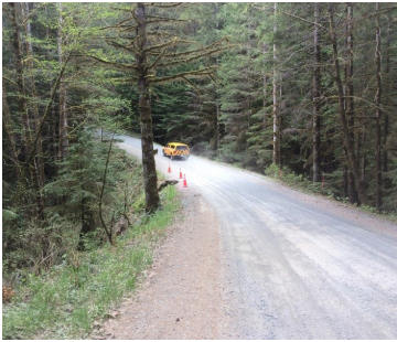
Loveland Bay Road – culvert crossing
