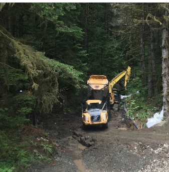
Instream work: aggraded material removed, new material added to reshape the channel
