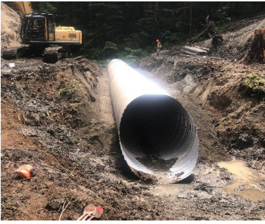
Original road crossing has been removed and culvert installation begins
