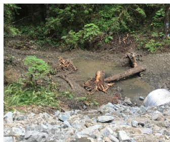
The finished product: Downstream view after channel restoration
