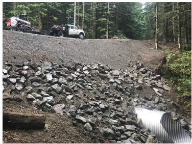
Road fill and riprap are added
