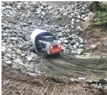
Culvert embedment process
