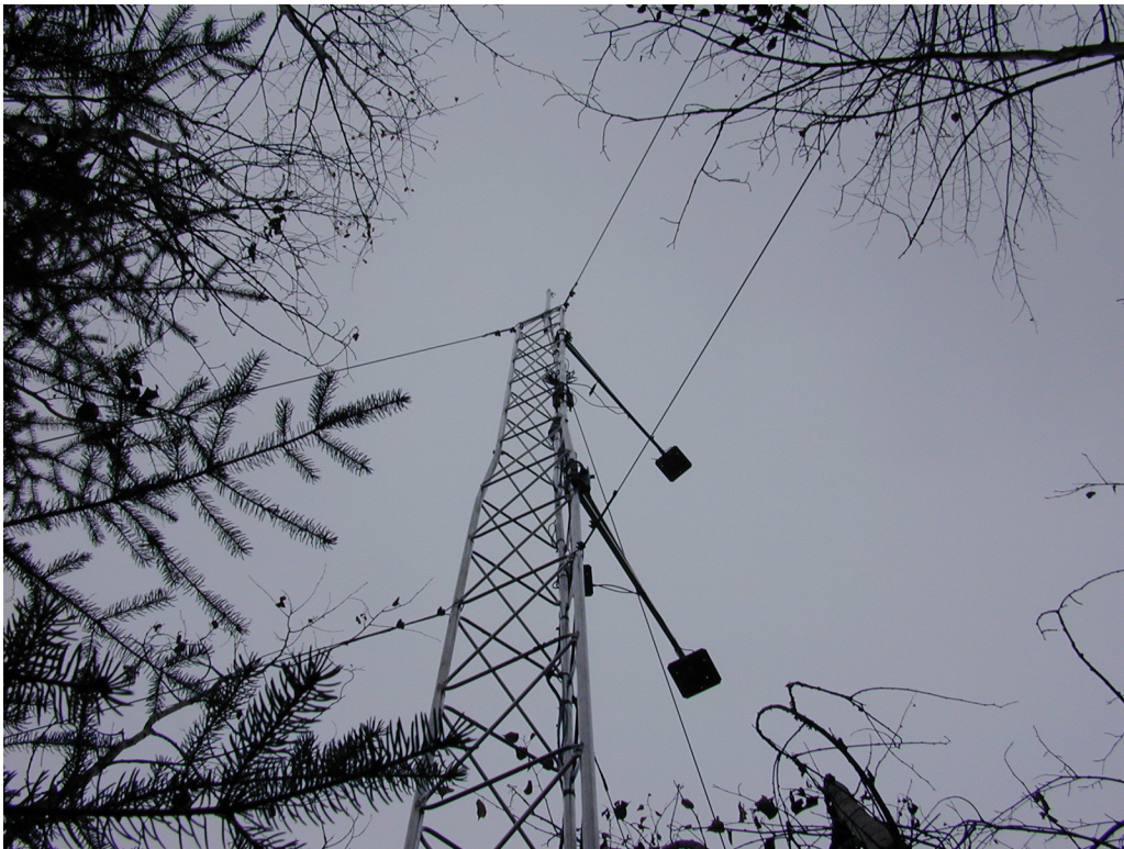
DSCN0673 Iron Creek Light Tower
