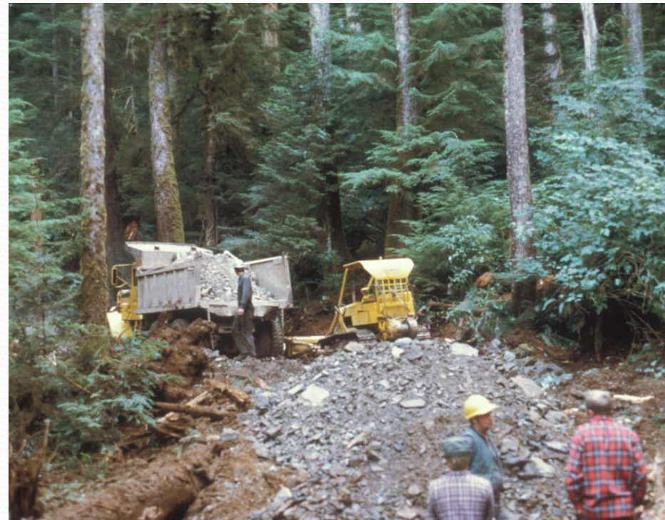
Road Construction in Carnation Creek, Aug 1971. Project photo.
