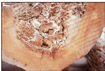
Brown crumbly rot decay with white mycelium.
