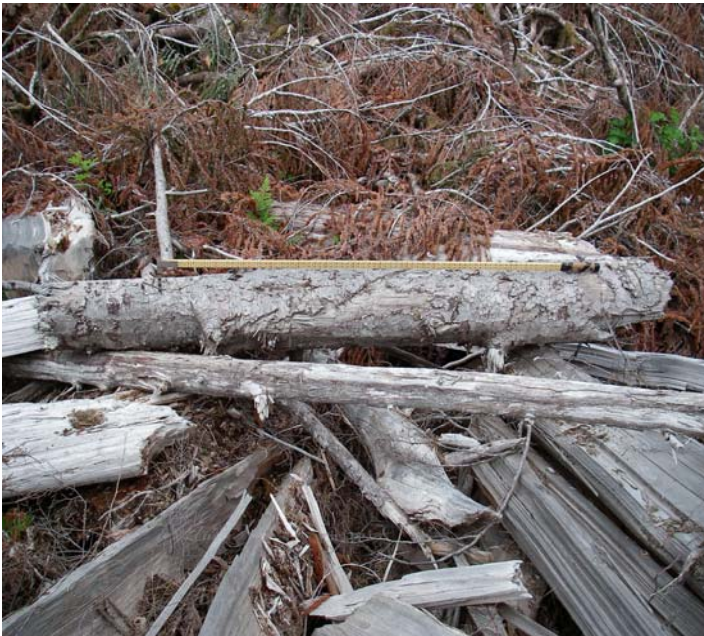
Broken butt, broken top & <3.0m
