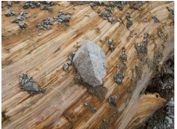
Imbedded rock in Cedar culvert log
