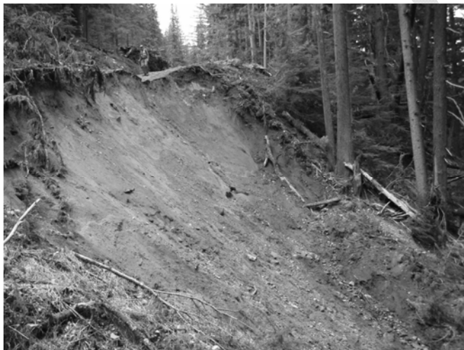
Figure 7. Debris slide of May 2008 below the Sitkum fire. The road is at the top of photo. Several holes from piping of groundwater are visible in the middle part of the slide scarp.
