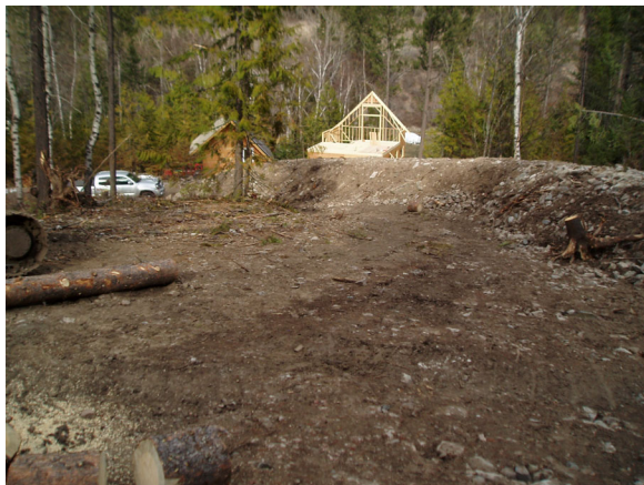
Figure 7. Mitigation works constructed to protect dwellings from increased debris flow hazard, Terrace Mountain fire. a) Constructing cross-ditches on abandoned logging road crossing gully. b) Berm on Wilson Creek fan. Photos: Tim Smith.
