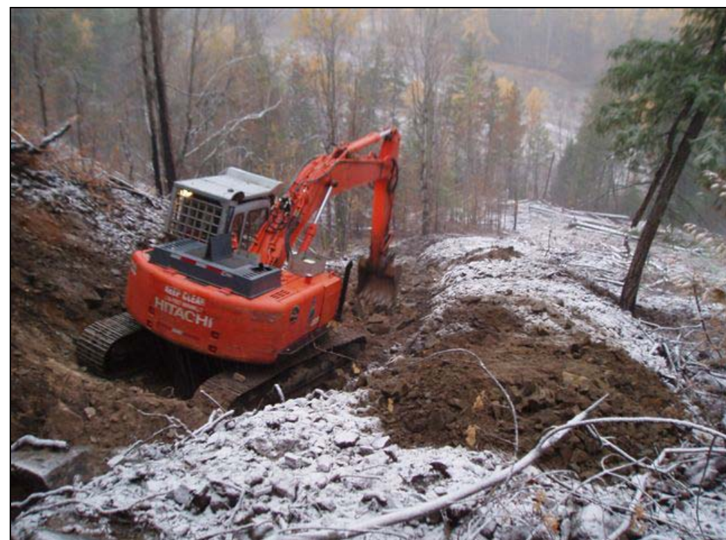
Berms constructed to protect houses from possible debris flows
