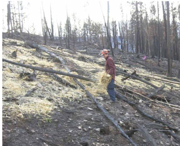
Spreading straw mulch by hand, Terrace Mtn fire, 2009
