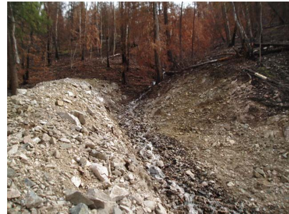
Berms to protect houses, Terrace Mtn fire, 2009
