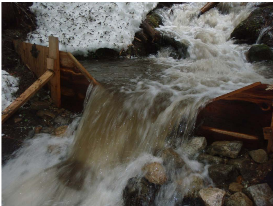
Sitkum T3 weir at peak flow
