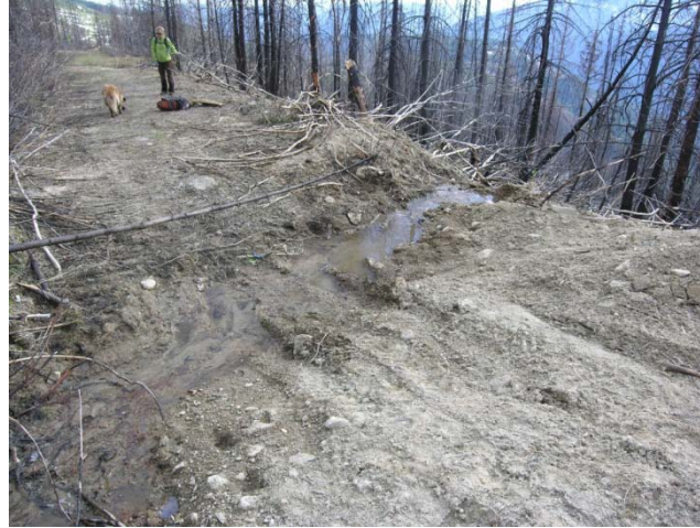
Cross-ditch, Springer fire
