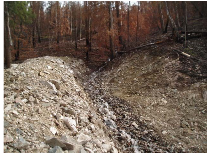
Berms and cross-ditches to protect houses, Terrace Mtn fire
