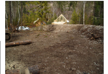
In late March of 2011, a small debris flow occurred in one of the gullies (left) during spring snowmelt. The berm successfully diverted the debris flow away from the house at the base of the slope.
