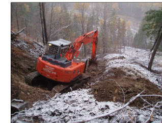
Berms constructed to protect houses from possible debris flows; October 2009.
