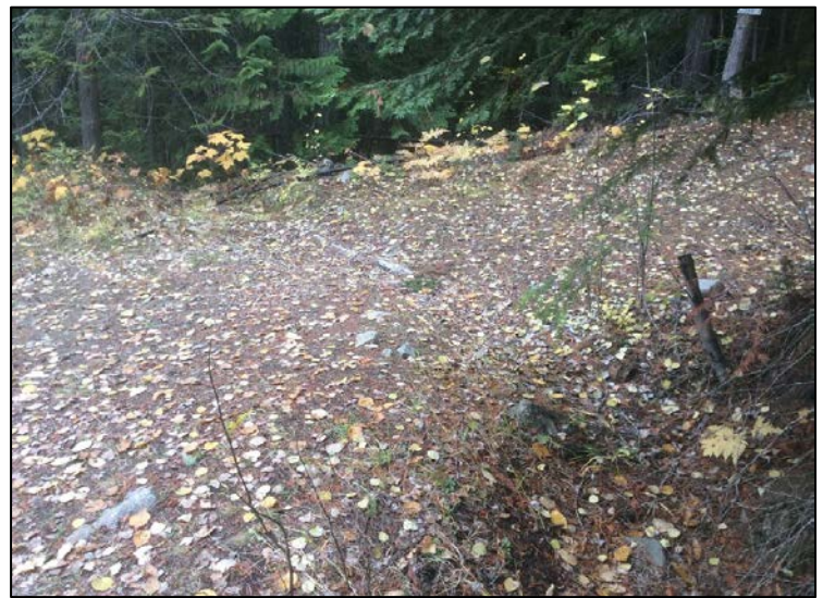
Image 15: looking downslope at the shallow cross-ditch at the start of the trail that heads west from the switchback of the private road (PM 30 on Figure 3).
