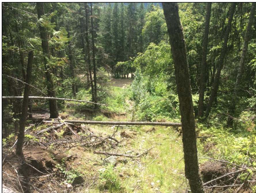
Image 3: View down the path of the debris slide that impacted Smallwood FSR approximately 5 years ago; the road is visible in the distance.
