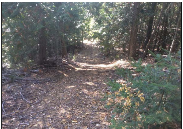
Image 5: looking southwest, down the existing trail in the northeast portion of Block 2. Outsloping of the trail presently prevents the significant redirection of runoff down the steep grade.
