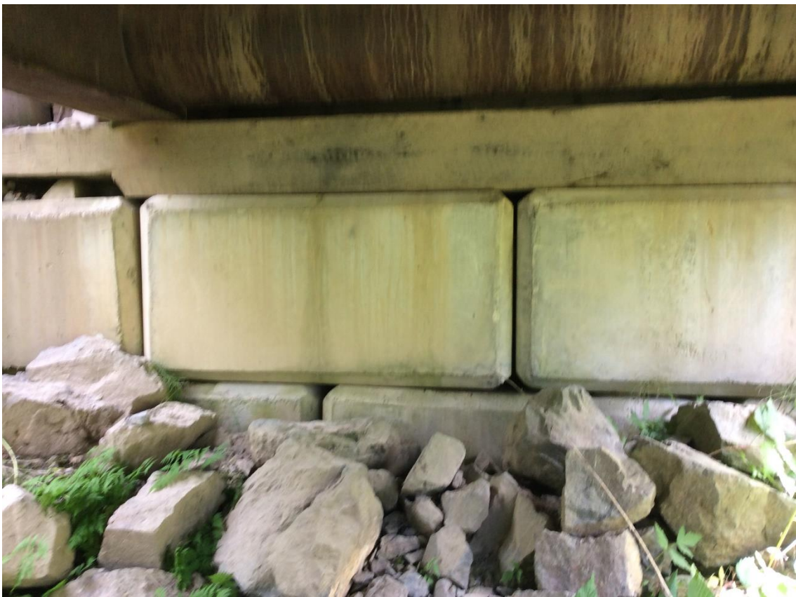
Structure G5-918 Lock Block Abutment
