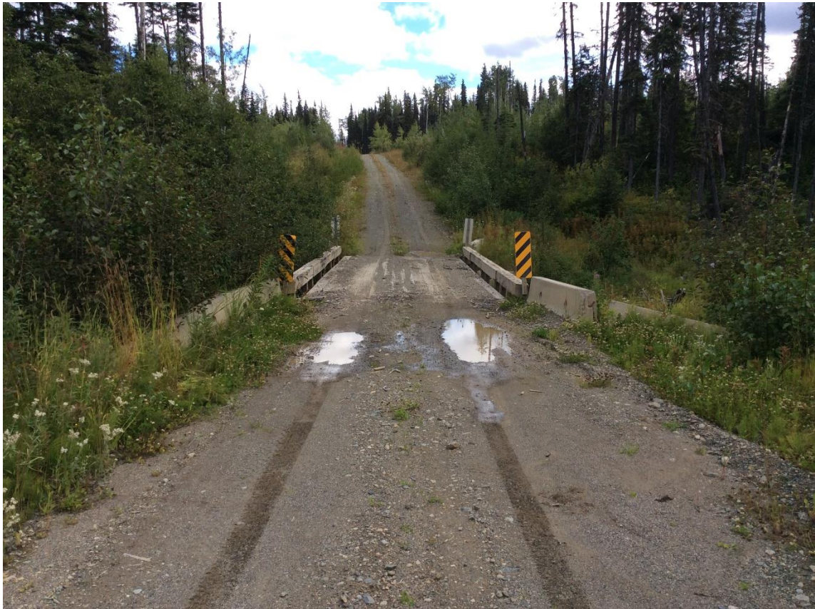
Structure G5-918 Facing Towards Bush
